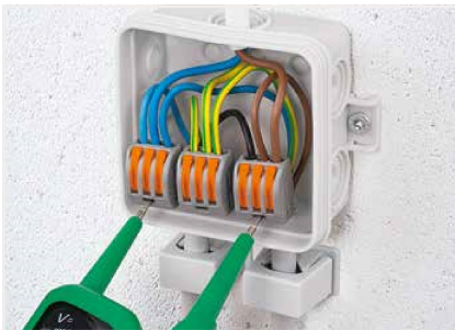
Testing the wired connectors
