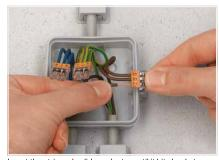
Insert the stripped solid conductor until it hits backstop.
